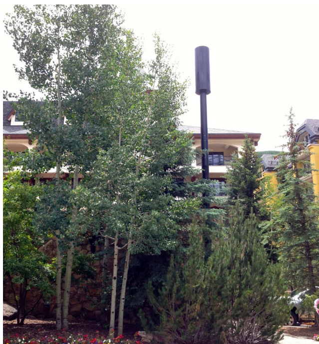
Figure 2: Actual Distributed Antenna System nodes within the Town of Vail
